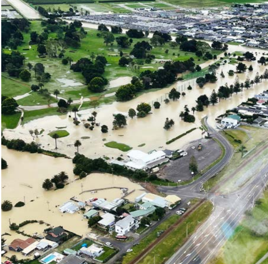
Flooding caused by Cyclone Gabrielle.
